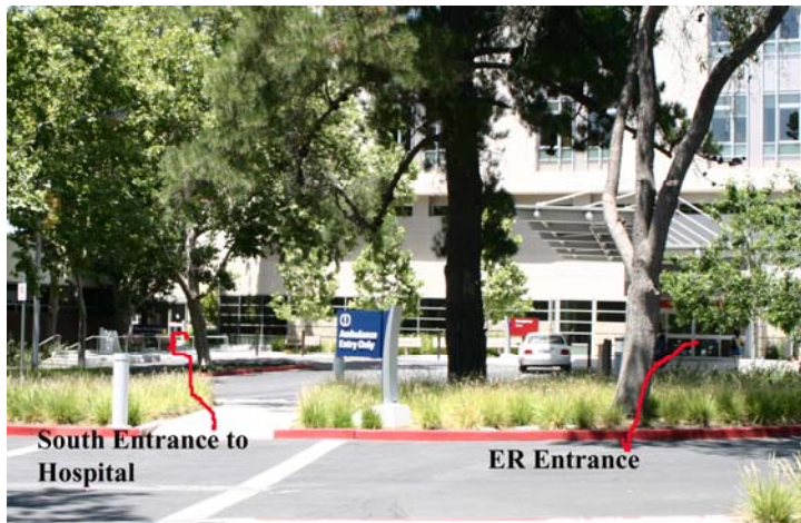
Figure 3: Emergency and South Entrances
