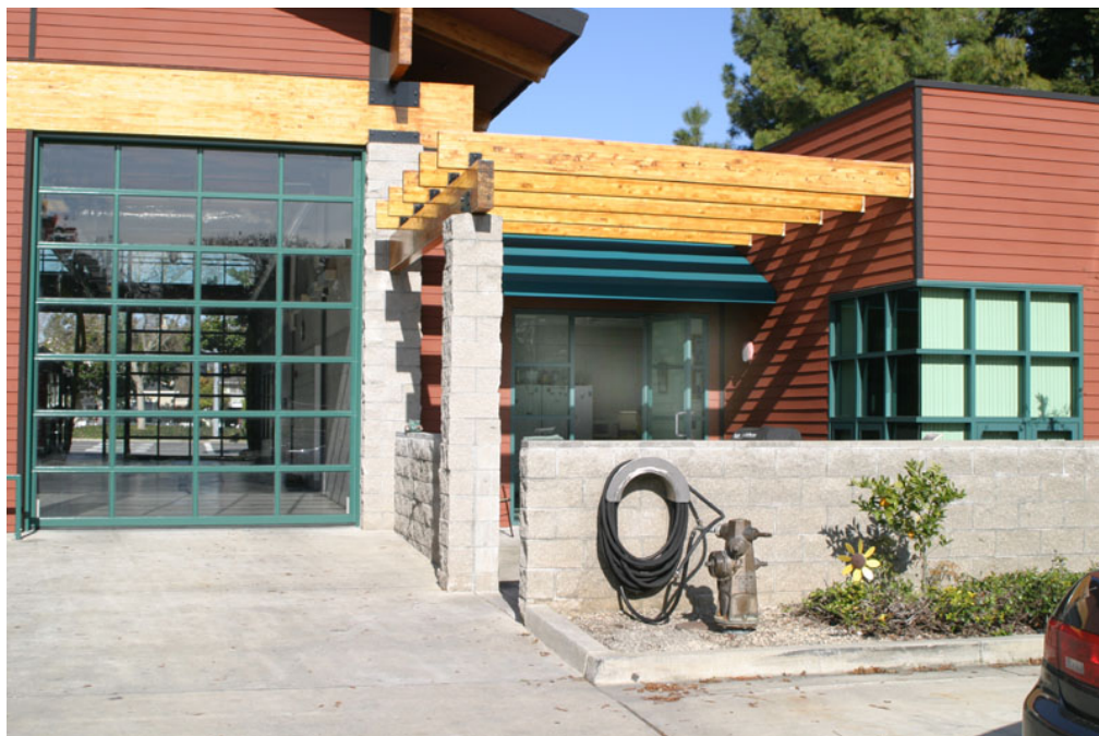
Photo FS1-1 – Rear Entrance to Fire Station 1
