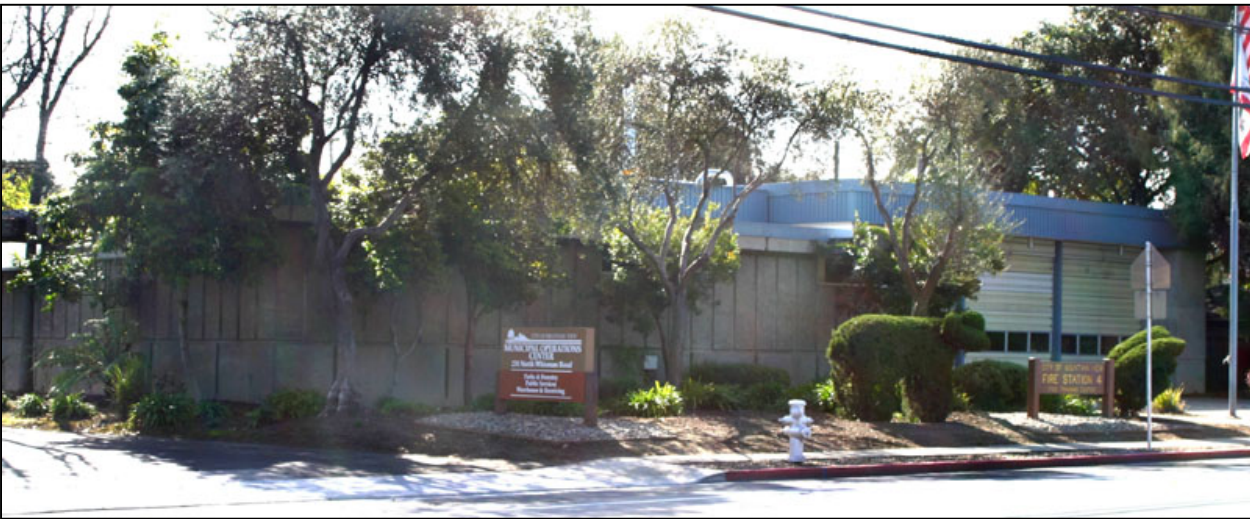
Photo FS4-1 – Fire Station 4 from Whisman Rd.
